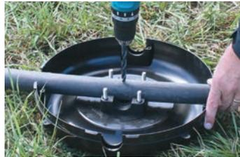
Drill 15mm (9/16") hole at required spacing for the sprinkler type being used and remove all drilling swarf. Ensure the hole is drilled perpendicular to the Pod Base. Caution: Do not drill through both edges of the pipe.
