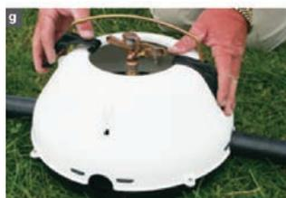
Fix wire clip into opposing holes on body sides. Ensure the wire runs parallel with the pipe as shown in the image.
