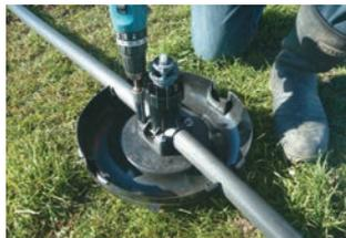
Fit O-ring seal to Pop-up Tapping Saddle Top, locate spigot into hole in pipe and fasten to Cross Tee Anchor, ensure fastening nuts are tightened evenly.
