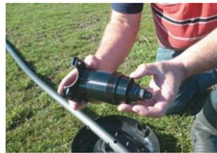
Screw either Nelson Mini Reg or Irripod ACME Male/Female High Riser onto ACME thread in base of Pop-up Piston and then place into Pop-up Tapping Saddle Top
