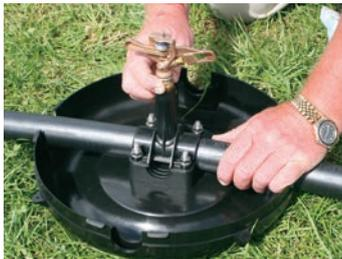
Screw sprinkler into sprinkler riser.
