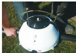
Locate Pop-up Pod Cover on top of Irripod Top Cover and ensuring the cutouts in the Pop-up Cover locate inline with the Pipe direction, fasten with screws.
