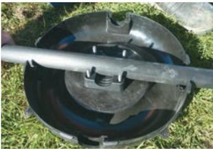
Lay pipe over Skid Base and secure in position with Cross Tee Anchor.
