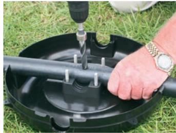
Drill 15mm (9/16") hole at required spacing for the sprinkler type being used and remove all drilling swarf. Ensure the hole is drilled perpendicular to the Pod Base.
