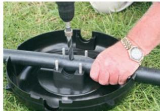
Drill 15mm (9/16") hole at required spacing for the sprinkler type being used and remove all drilling swarf. Ensure the hole is drilled perpendicular to the Pod Base.
