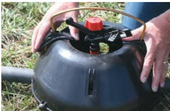
Fix wire clip into opposing holes on body sides. Ensure the wire runs parallel with the pipe as shown in the image.
