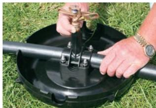
Screw sprinkler into sprinkler riser.
