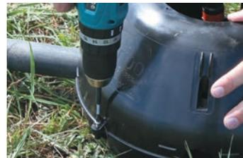
Secure top body by screws around the base.
