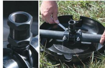
Fit O-ring seal to the under side of Riser. Screw the 20mm Hansen Socket onto the Riser thread and locate riser spigot into hole in pipe. Tighten nuts evenly to fasten the cross tee anchor and tighten socket.
